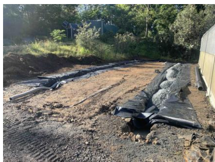
Installing drainage
